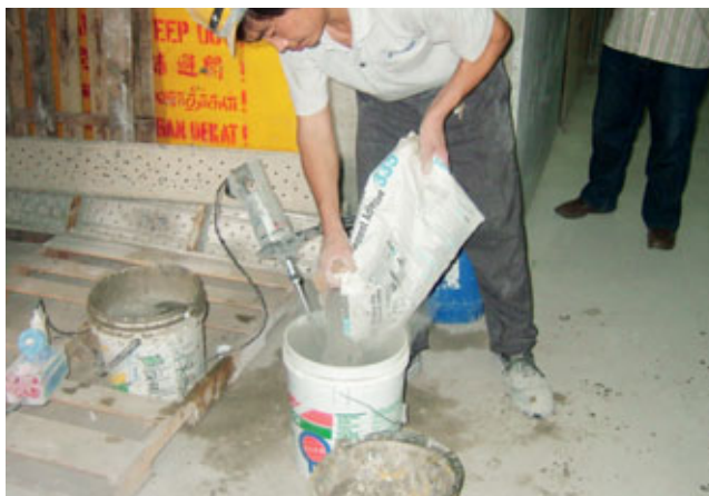
Fig. 5.7 – 1-component adhesive: Add powder + clean potable water.
